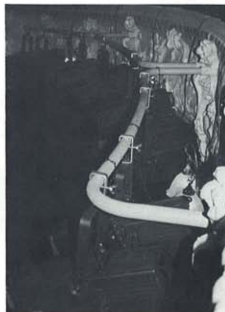
Lighting bars fixed to tier fronts are easily removable - the auditorium can be returned to a totally 'clean' state with a minimum of fuss.
