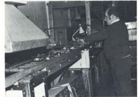
Flow soldering in action.
